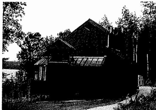
6. Holiday Home, Killykeen Forest Park, Co. Cavan 1986, Architect: Ciarán O'Connor, OPW
